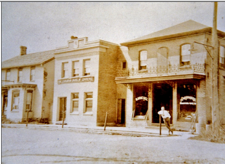
The Hardware Store of Bert Kriesel c. 1908 from the Wilmot Township Archives.
