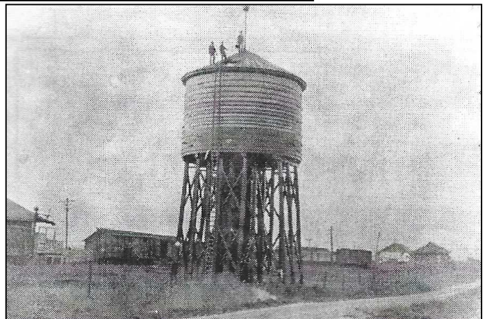
Grand Trunk Water Tower, Charlotta Street, Baden
