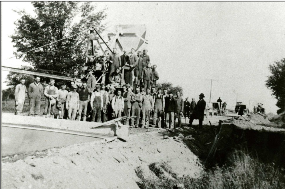
Photo: Highway Construction in New Hamburg, Township of Wilmot Archives
