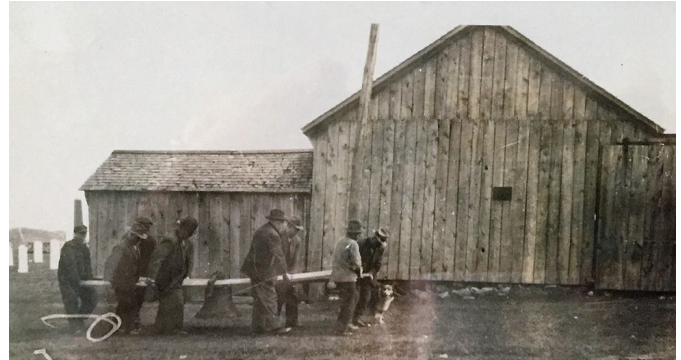
Men carrying the bell to be installed in the new church which was built in 1929.
