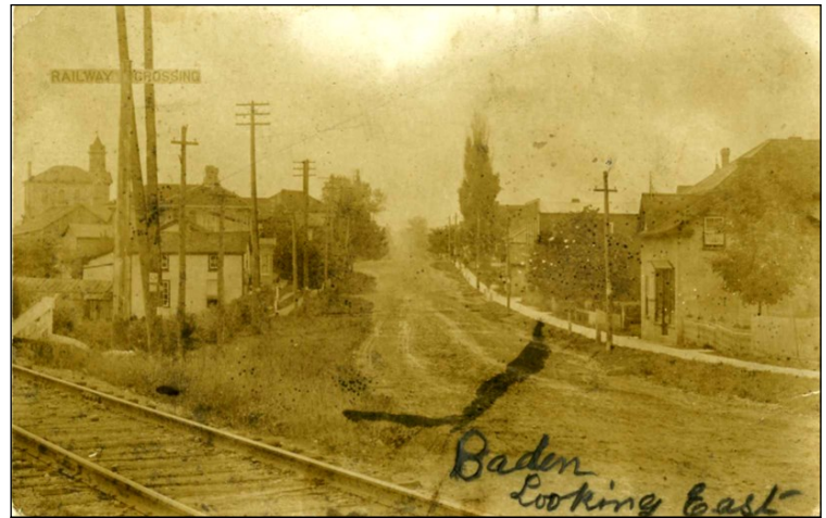
Utility poles on Snyder’s Road East in Baden c.1910s.
