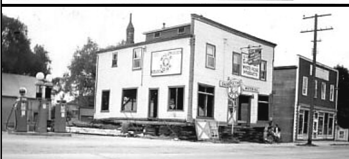
The garage in early 40s is jacked up on logs and ready to move.
