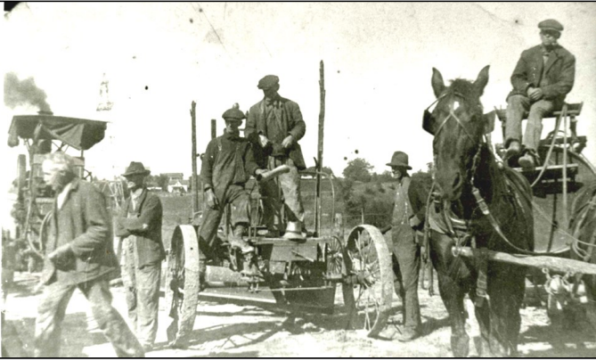
Photo: Road work in Wilmot. Township of Wilmot Archives
