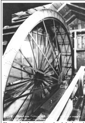
The undershot waterwheel designed and built by Abraham Gingerich
