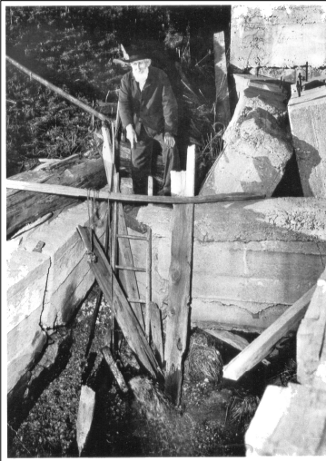
Abraham pointing out his turbine amongst the ruins of his power generating building
